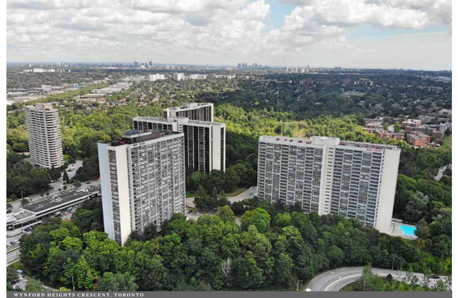
WYNFORD HEIGHTS CRESCENT, TORONTO
