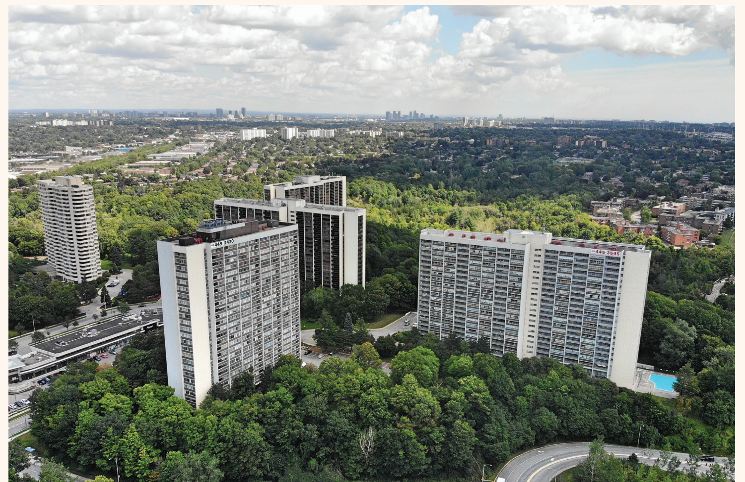
Wynford Heights Crescent, Toronto
